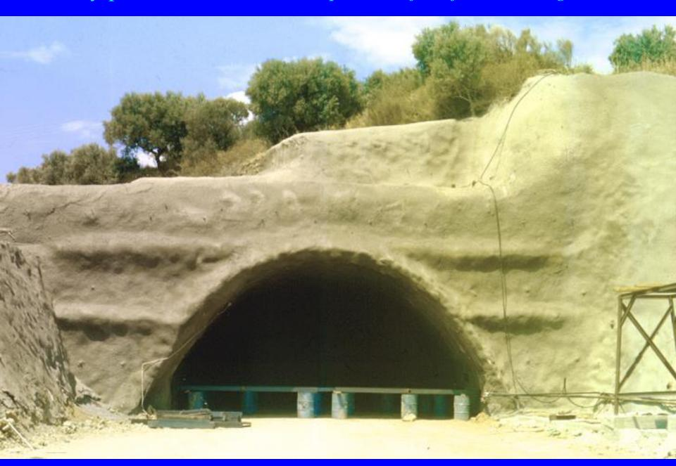
Patra by-pass road tunnel - South portal failure - August 1998
