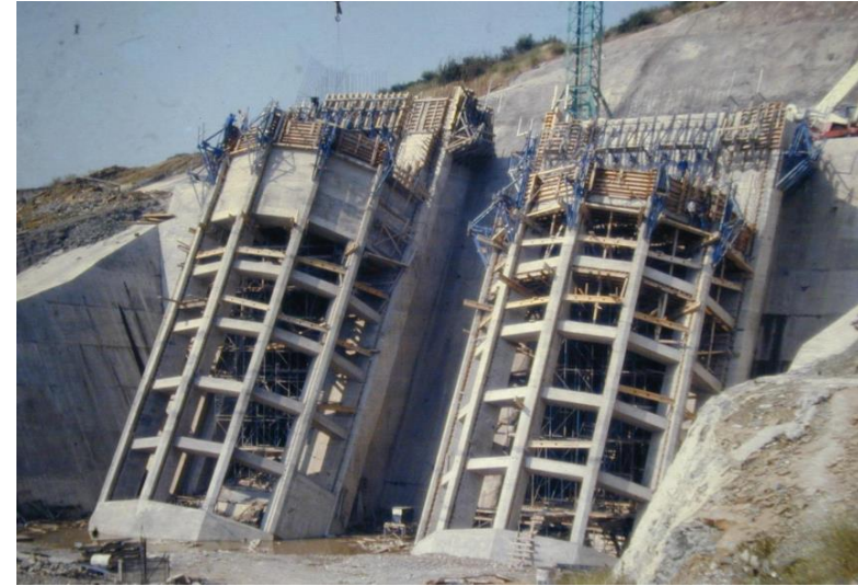
Stratos dam: inclined intakes under construction
