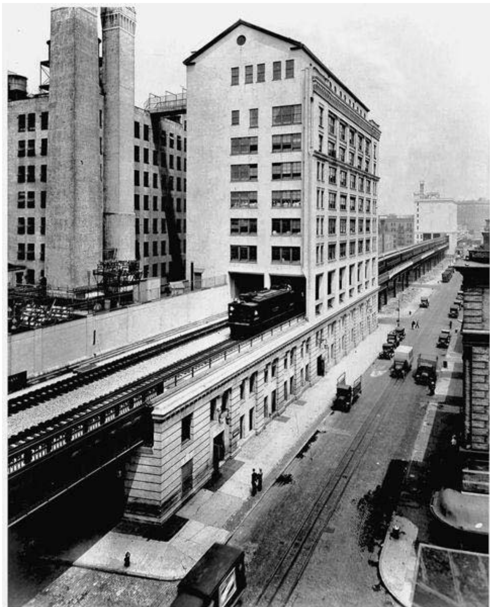
THE WEST STREET HEADQUARTERS OF BELL LABORATORIES, WITH TRAINS OF THE HIGH LINE RUNNING THROUGH
